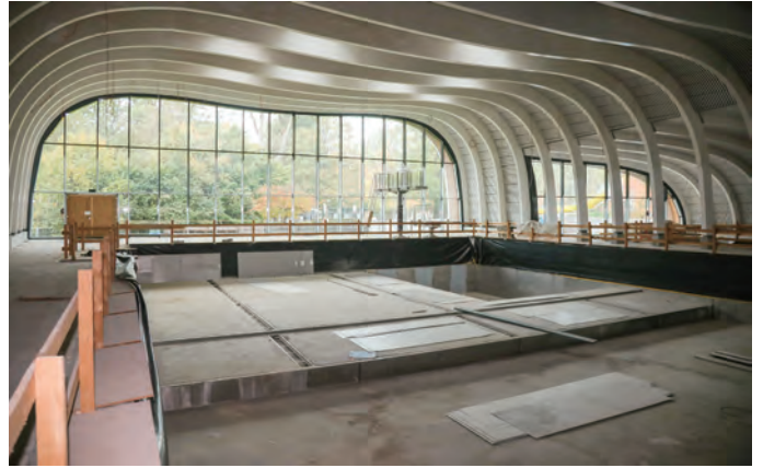
Hallenbad Dachau (Dachau, Germany) (建設中)
